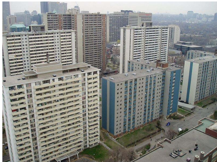
Figure 2. St. Jamestown Public Housing in Toronto
